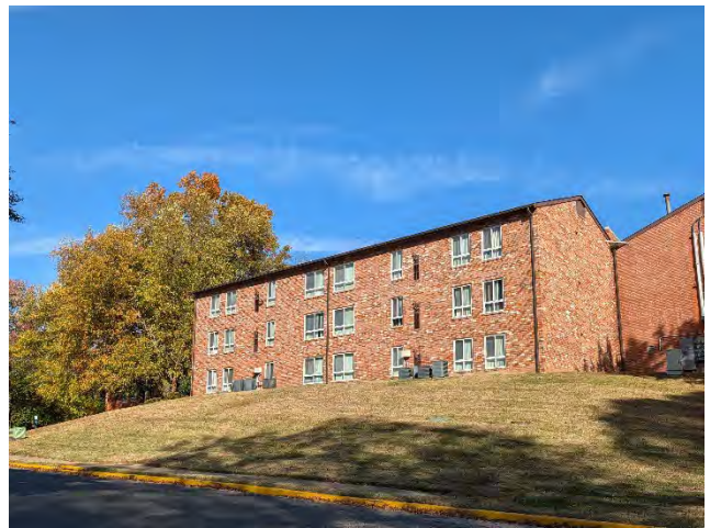
Multifamily to the Northwest
