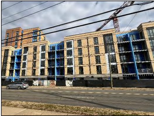
Phase I southwest of site from W Glebe Rd
