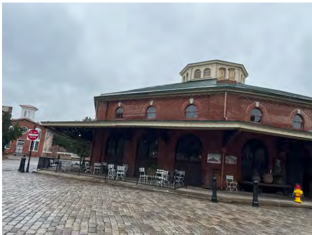
Commercial use to the north of the Subject
