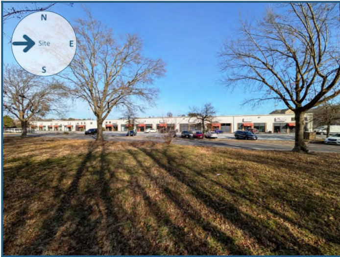
View of site from the west
