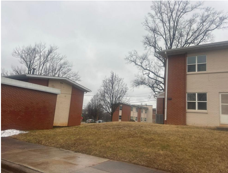
View to the North
