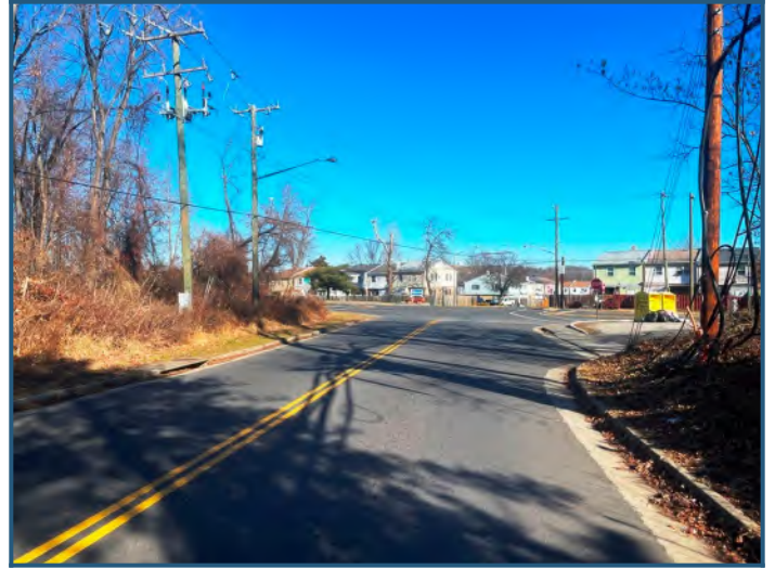
Streetscape: North view of Old Triangle Road
