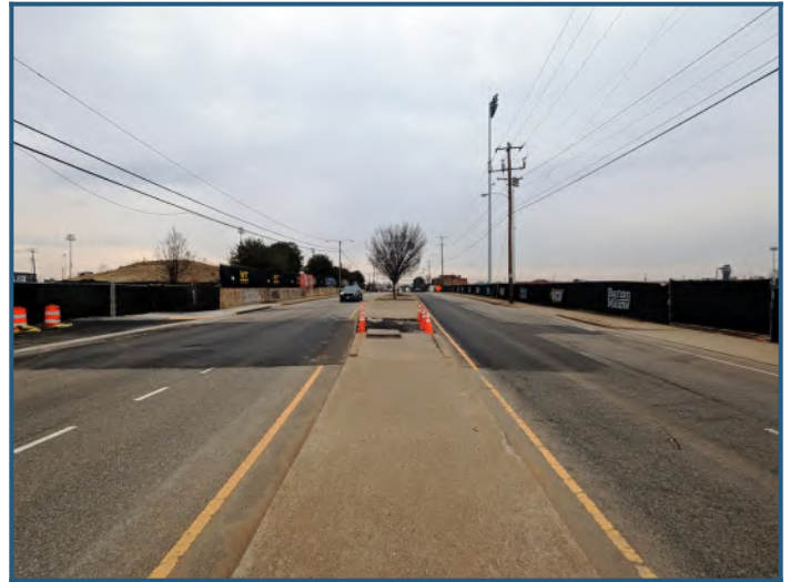
Streetscape: North View of Hermitage Road
