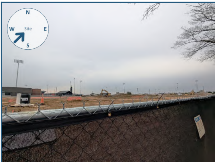
View of site from the southwest
