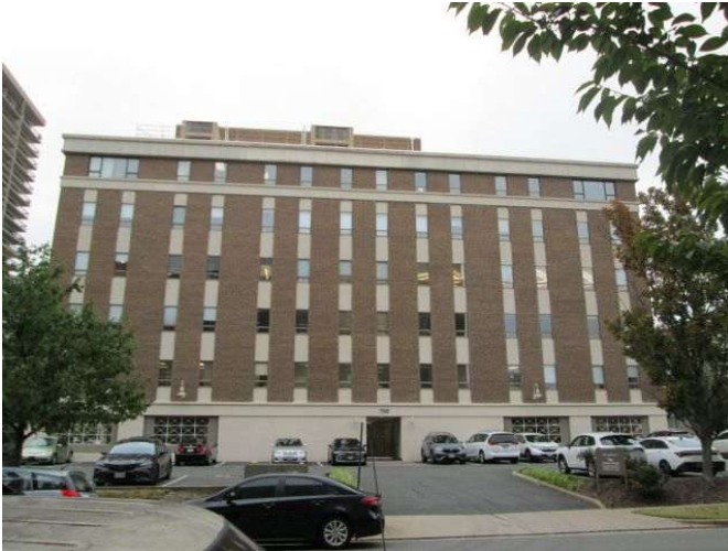
Office building north of the Subject
