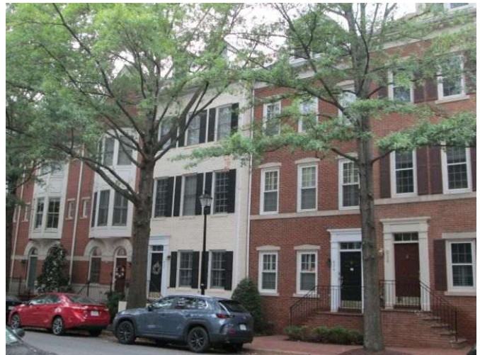
Owner owned townhomes west of the Subject site
