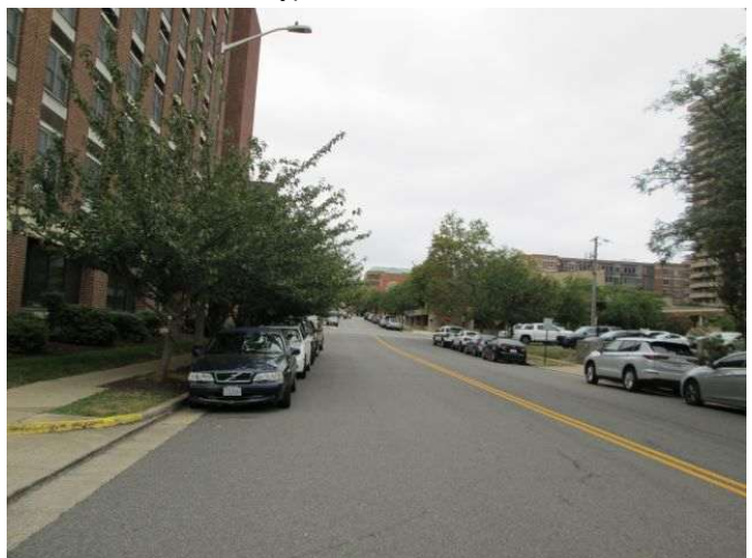
View west along Wythe Street
