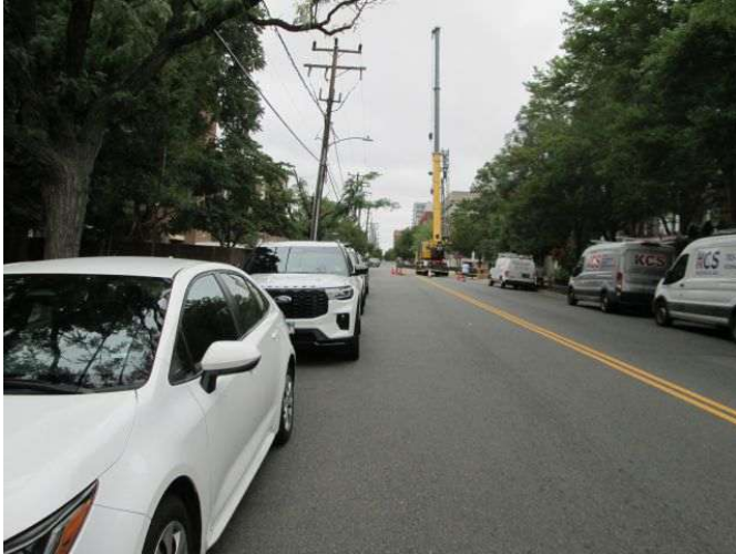
View north along North Fairfax Street
