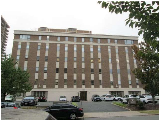
Office building north of the Subject
