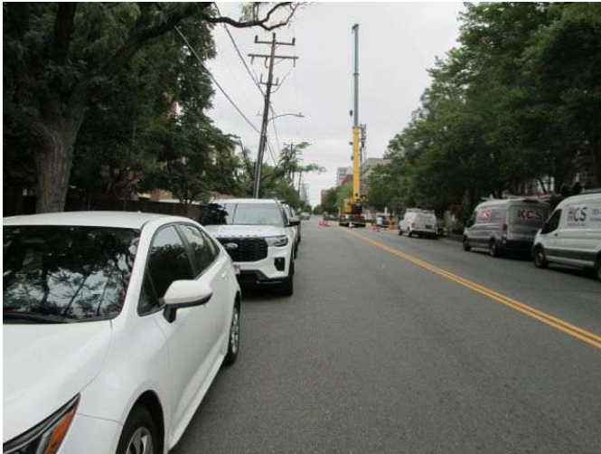
View north along North Fairfax Street
