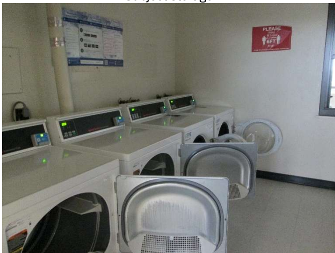
Subject central laundry facility
