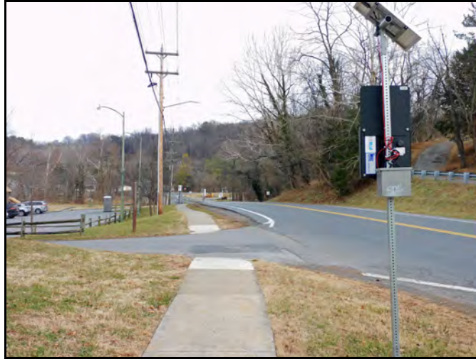
View east on E Criser Rd., at entrance to site
