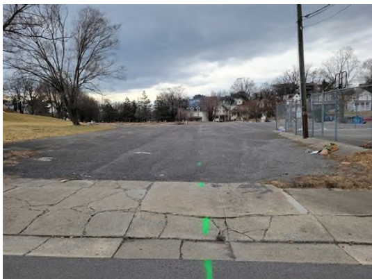
View of existing entrance to site on 7 th St facing west
