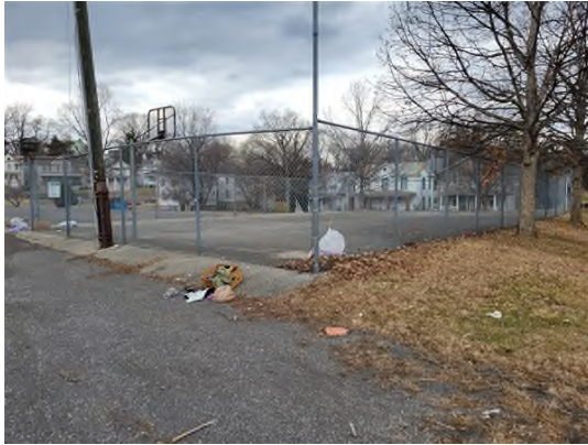
View of fenced basketball court on the site
