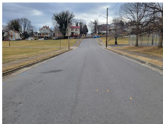
7 th St splitting the site
