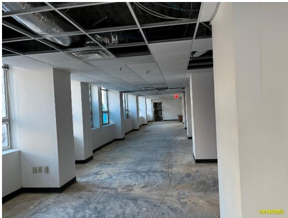
Partially Rehabbed Common Area
