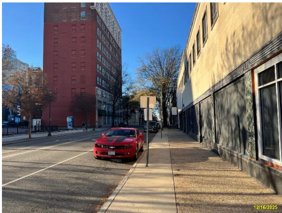
North 4 th Street Facing South
