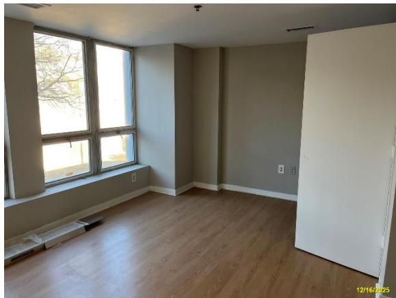
Partially Rehabbed Unit Living Area
