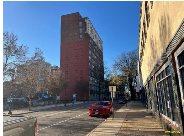
Subject Building (Rear) and Parking Area
