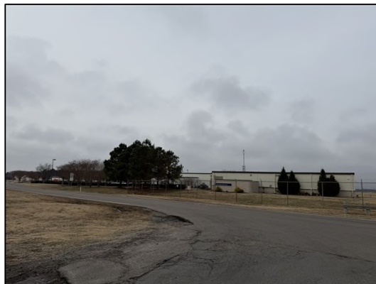
Industrial facilities beyond Miller Store Rd north of site
