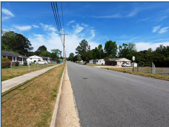
Streetscape: North view of Banks Street
