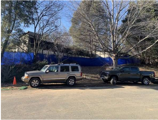
View of site facing northwest from Premier Circle
