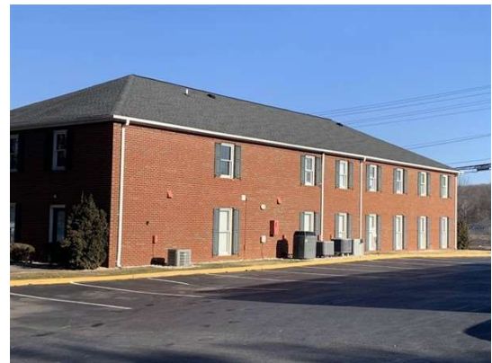
Office building east of site along Premier Circle
