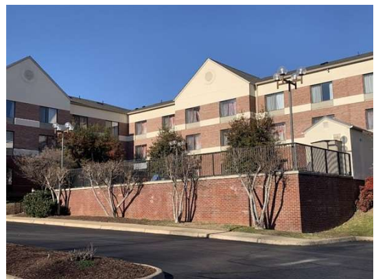
Hotel east of site along Route 29/Seminole Trail
