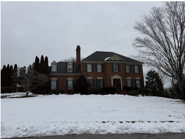
Typical single-family home west of Subject
