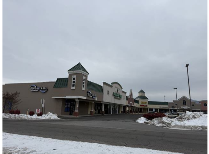
Commercial west of Subject site
