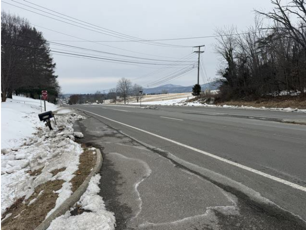
View of Williamson Road facing southwest
