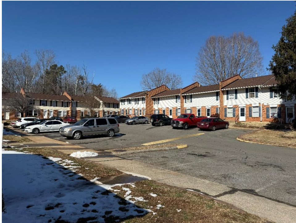
View of Parking
