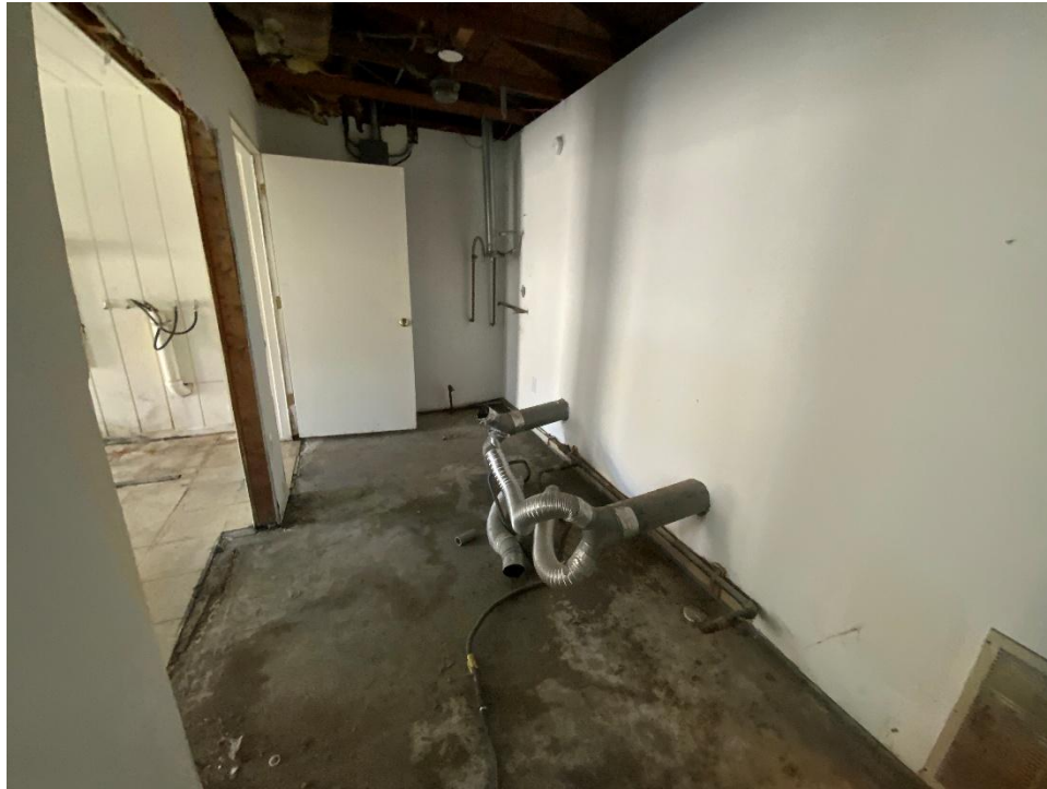
View of Laundry Facility
