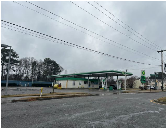
Gas station/convenience store south of Subject site
