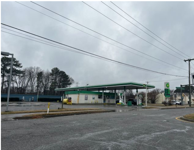
Gas station/convenience store south of Subject site
