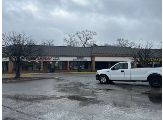
Retail center immediately south of Subject site
