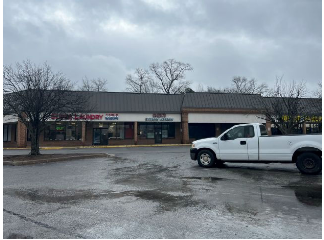
Retail center immediately south of Subject site
