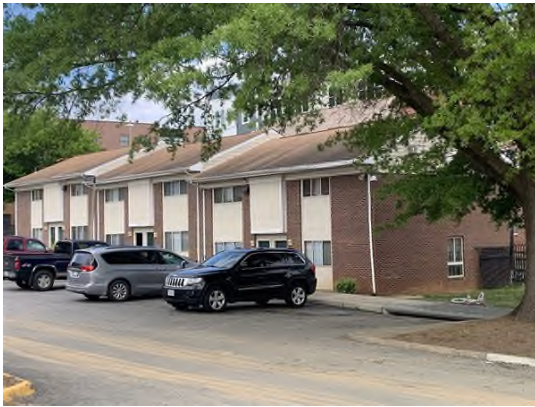
Existing Friendship Court structures north of site
