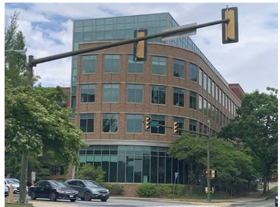
Office building west of site along 2 nd Street SE
