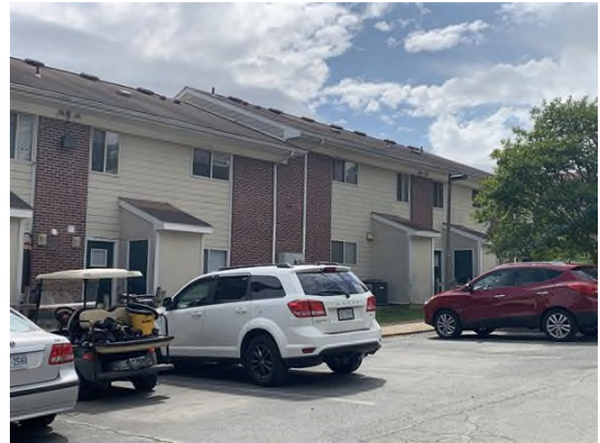
View of site facing southwest
