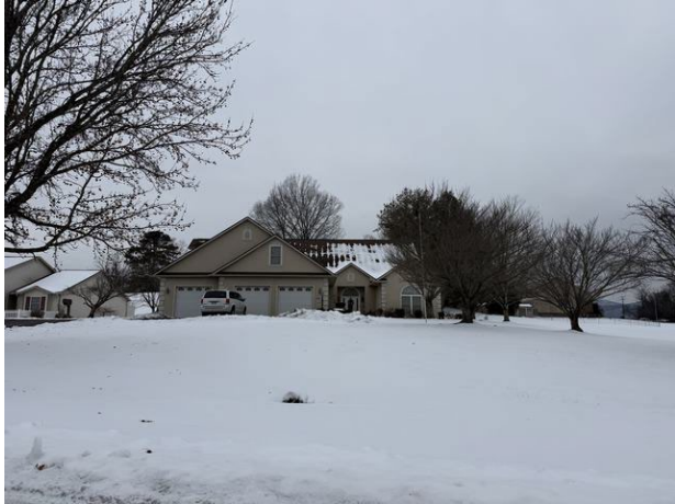
Typical single-family east of Subject
