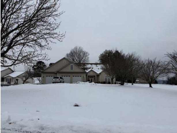
Typical single-family east of Subject
