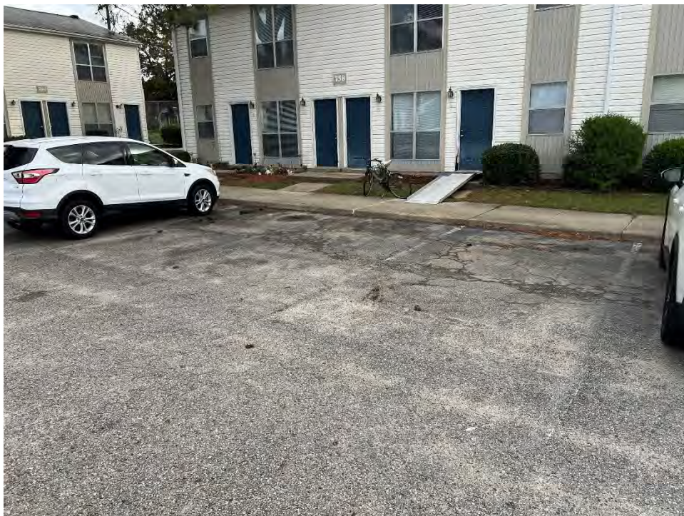
View of Parking
