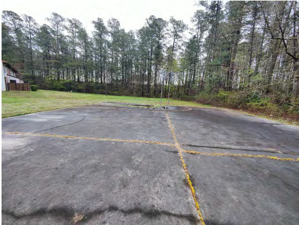
View of Basketball Court
