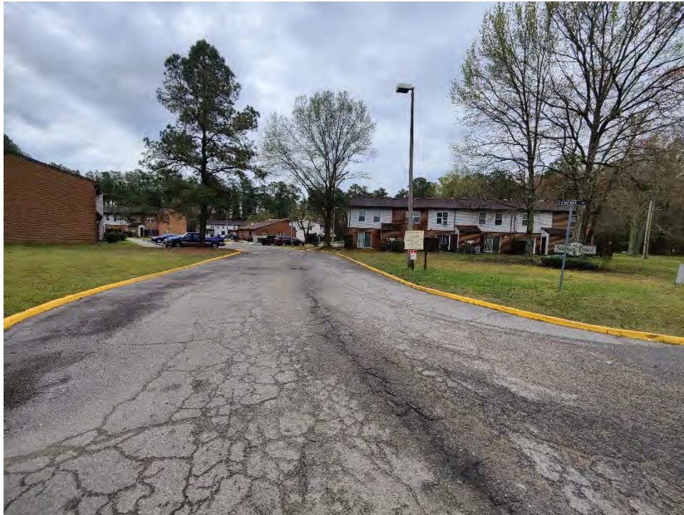
View of Entrance
