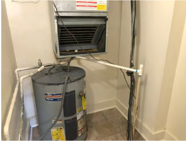
Typical mechanical area - vacant unit
