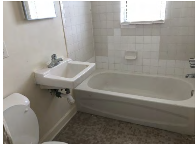
Typical bathroom – vacant unit
