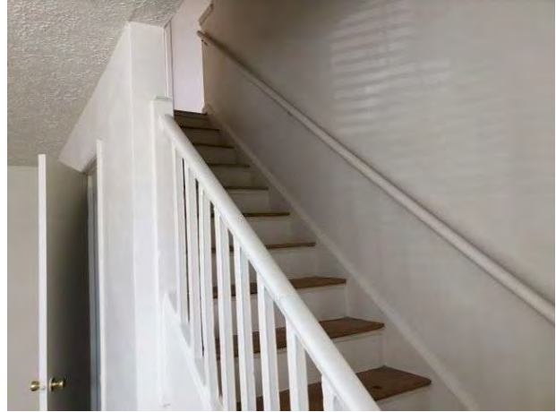
Typical interior stairway – vacant unit
