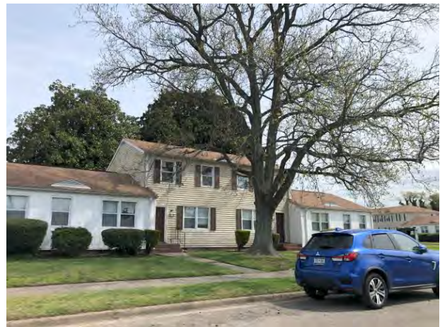
Typical Subject building
