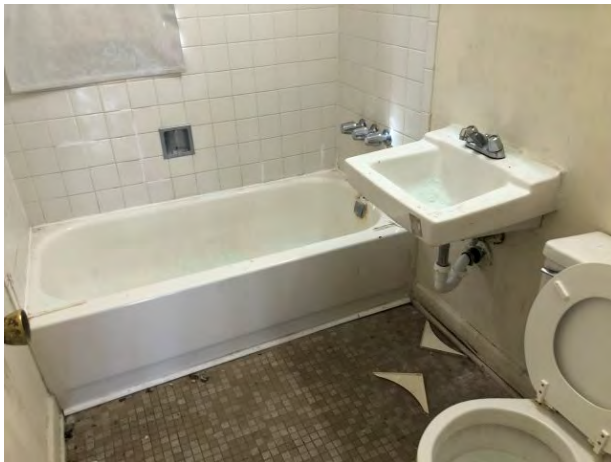
Typical bathroom – vacant unit
