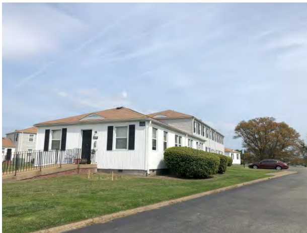
Typical Subject building
