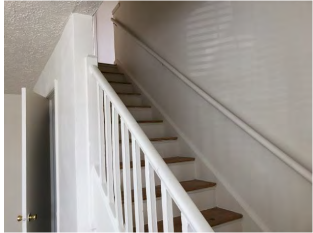
Typical interior stairway - vacant unit
