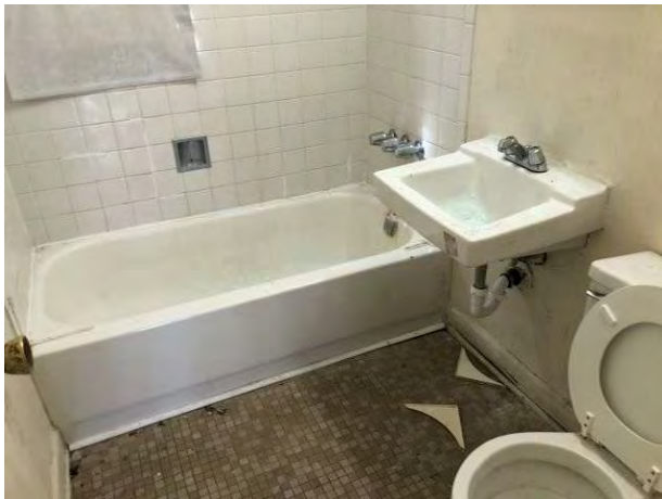
Typical bathroom – vacant unit
