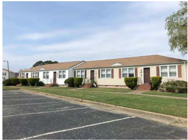
Typical Subject building
