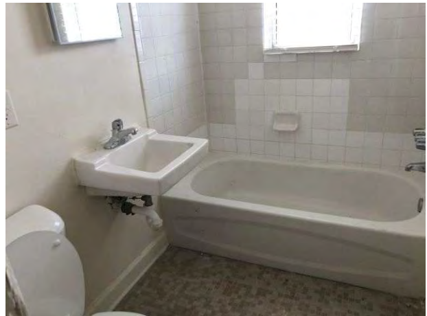
Typical bathroom – vacant unit
