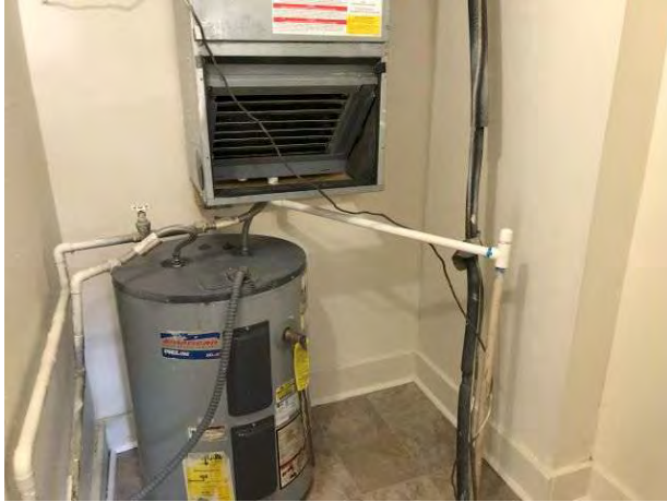
Typical mechanical area – vacant unit
