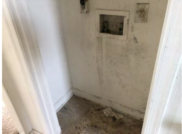
Typical washer/dryer connection area – vacant unit
