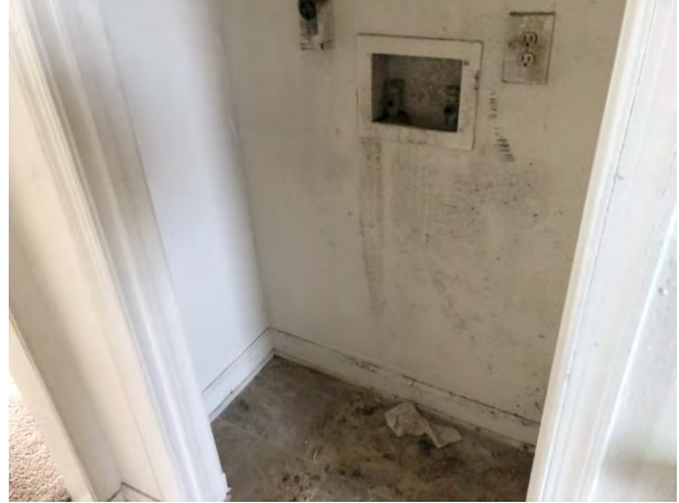
Typical washer/dryer connection area - vacant unit
