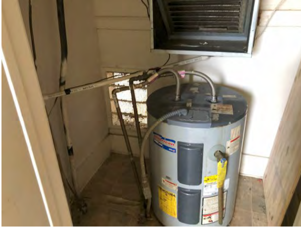
Typical mechanical area - vacant unit
