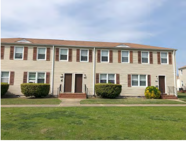
Typical Subject building
