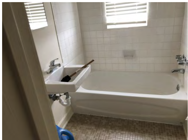
Typical bathroom – vacant unit
