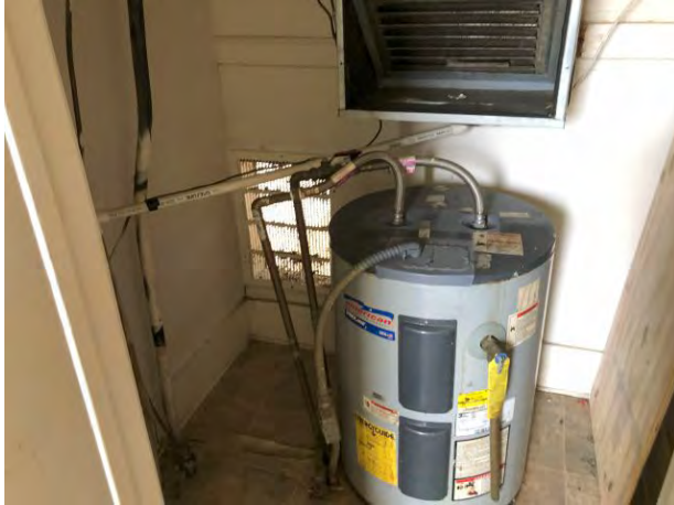
Typical mechanical area – vacant unit
