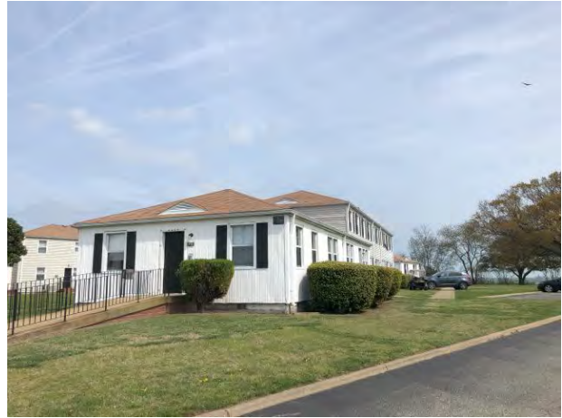
Typical Subject building
