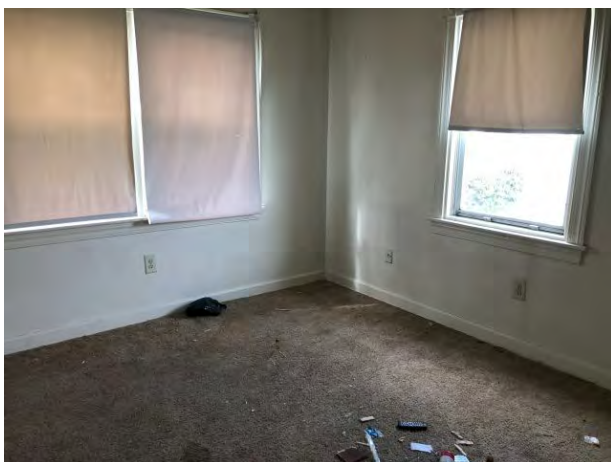
Typical living area – vacant unit
