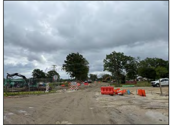
View of site (beyond construction) facing east from Chapel St
