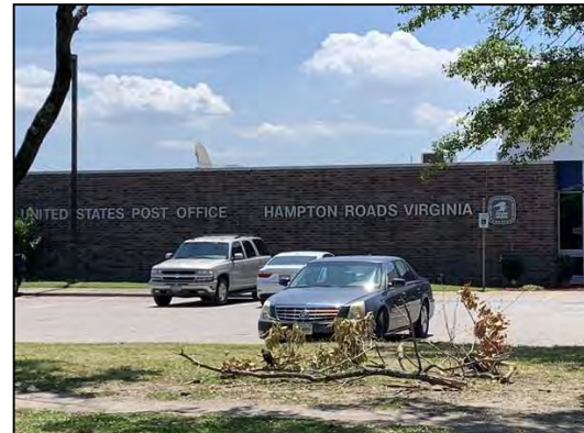
Hampton Roads Post Office, north of site
