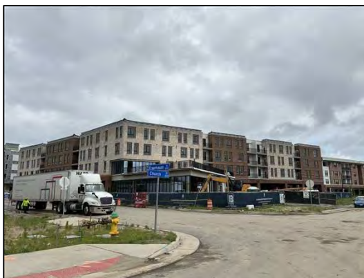
Unity Place Apartments under construction west of site
