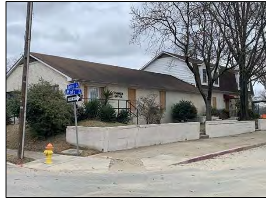
Church office adjacent to the site at the intersection of Reilly Street and Holt St
