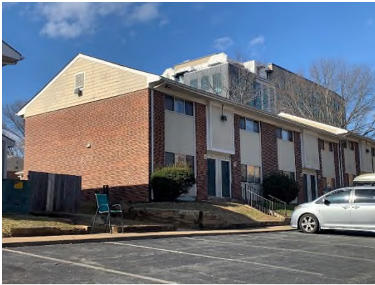
Existing Friendship Court structures north of site
