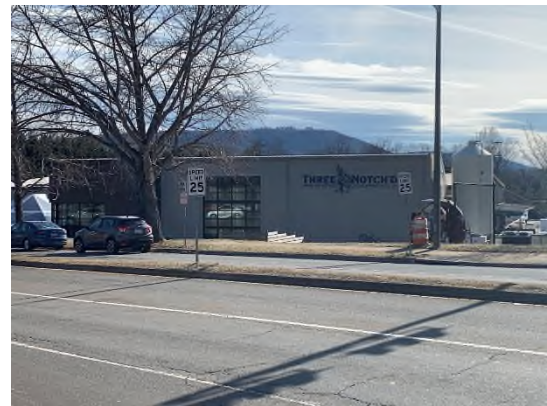
Three Notched Brewery south of site along Monticello Ave
