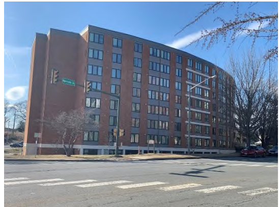
Office building southwest of site along Monticello Ave
