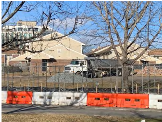
View of site facing north from Monticello Avenue
