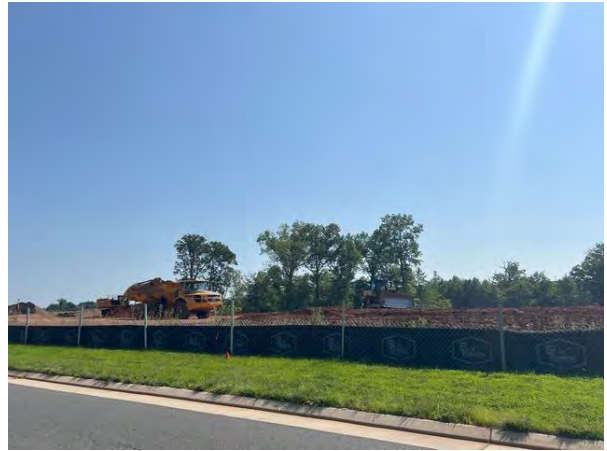
Avonlea Senior Phase I under construction directly east of the Subject site
