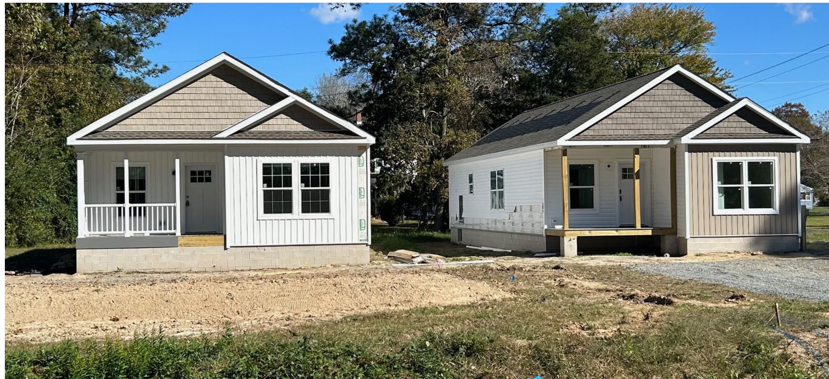
Accomack County, in partnership with iUnit Communities, built two Net Zero-Ready modular cottages.
