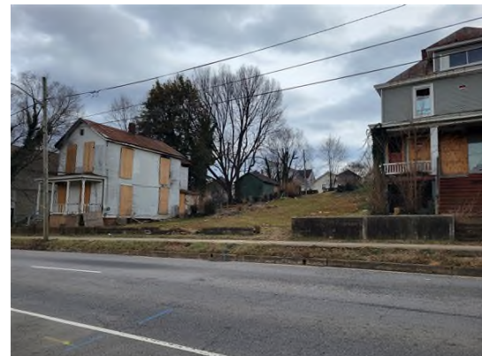
Vacant single-family homes/vacant lot fronting Bullitt Ave south of site
