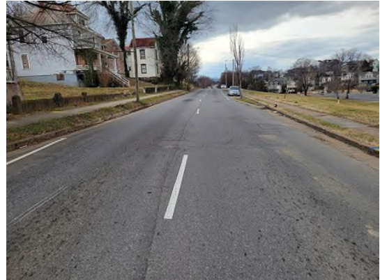
Bullitt Ave south of site
