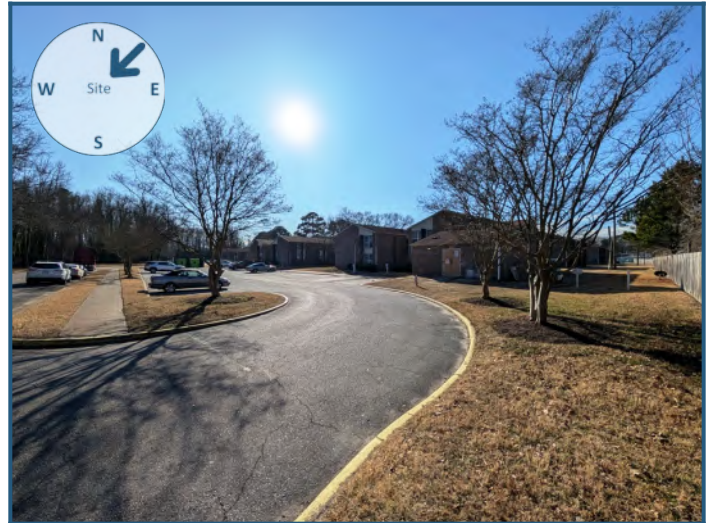
View of site from the northeast
