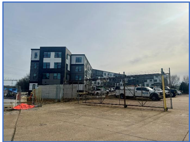
Spur Line Lofts
