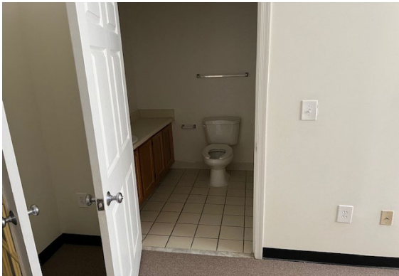
Typical Unit Interior
