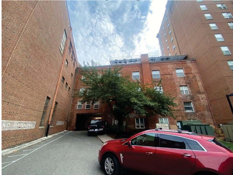
Rear Building, Parking Lot View
