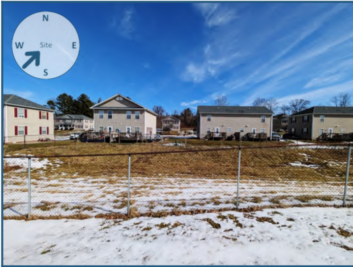
View of site from the southwest
