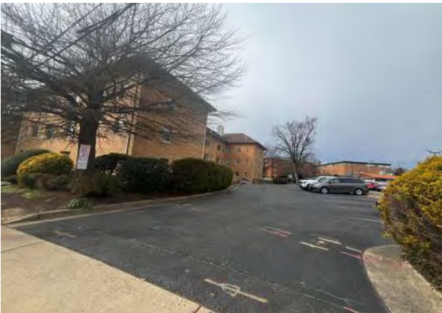
Subject site (existing improvements to be demolished)
