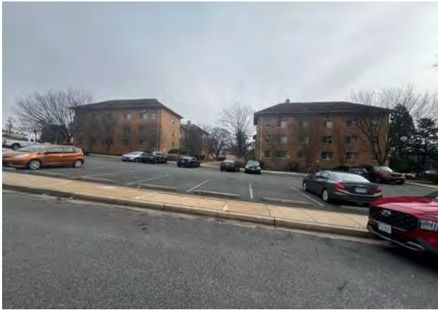
Subject site (existing improvements to be demolished)
