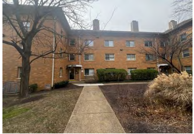
Subject site (existing improvements to be demolished)
