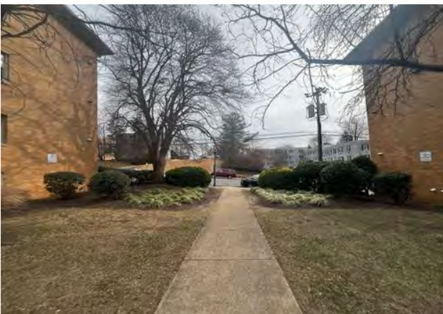
Subject site (existing improvements to be demolished)
