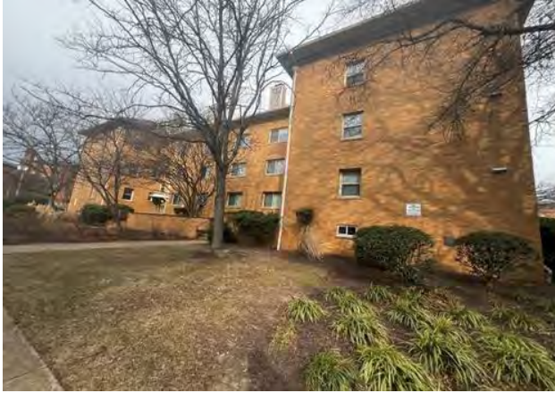
Subject site (existing improvements to be demolished)
