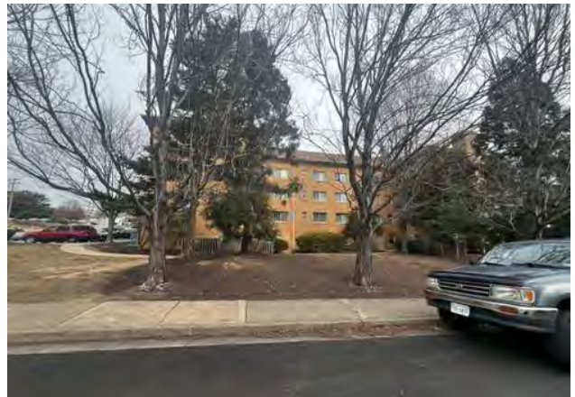
Subject site (existing improvements to be demolished)
