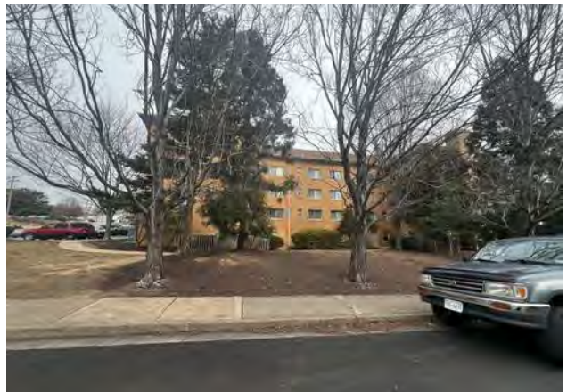
Subject site (existing improvements to be demolished)
