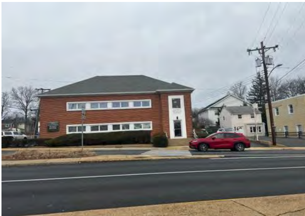
Commercial uses west of the Subject site
