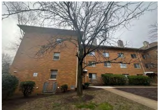
Subject site (existing improvements to be demolished)
