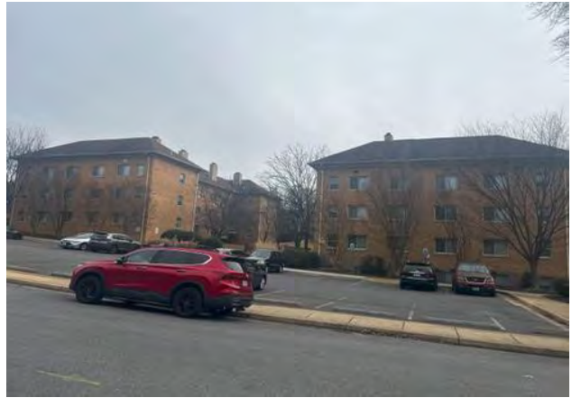
Subject site (existing improvements to be demolished)
