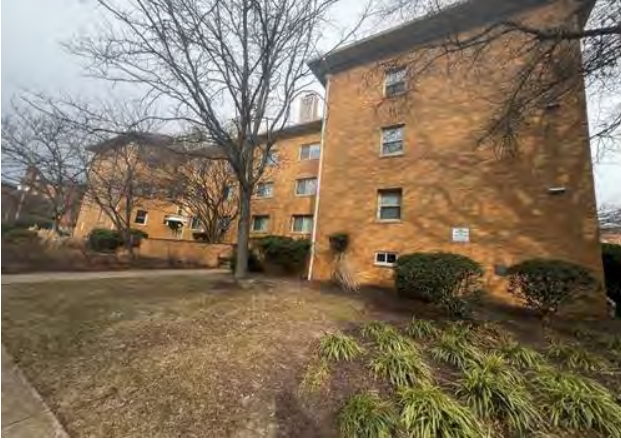
Subject site (existing improvements to be demolished)
