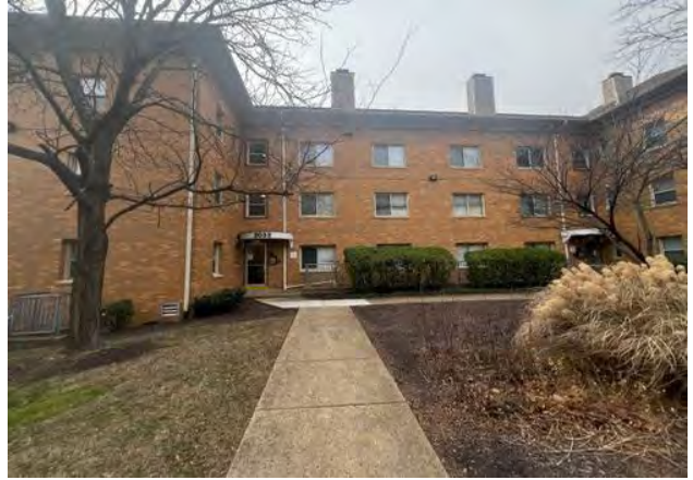
Subject site (existing improvements to be demolished)
