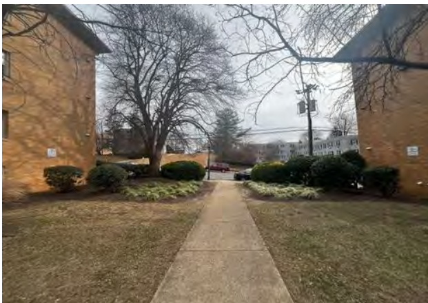
Subject site (existing improvements to be demolished)
