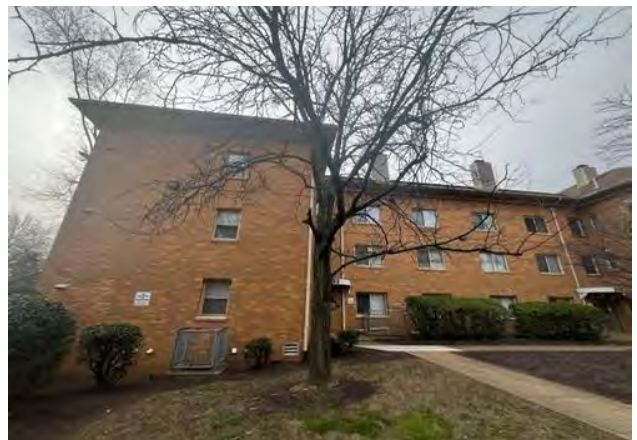
Subject site (existing improvements to be demolished)
