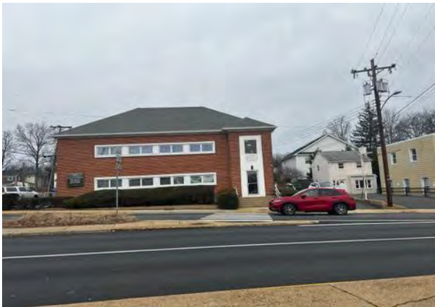
Commercial uses west of the Subject site
