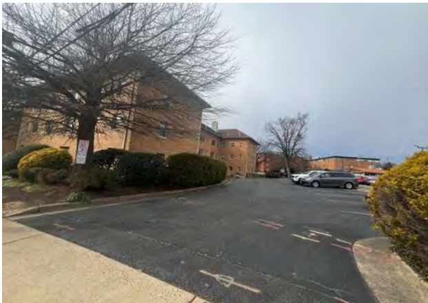
Subject site (existing improvements to be demolished)
