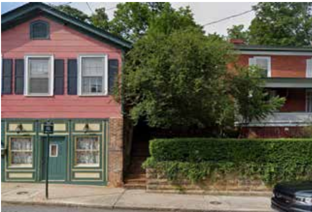
Looking North From Entrance
