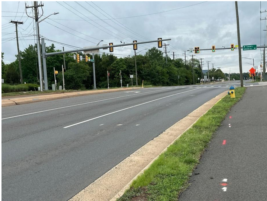
View Northwest on Godwin Drive
