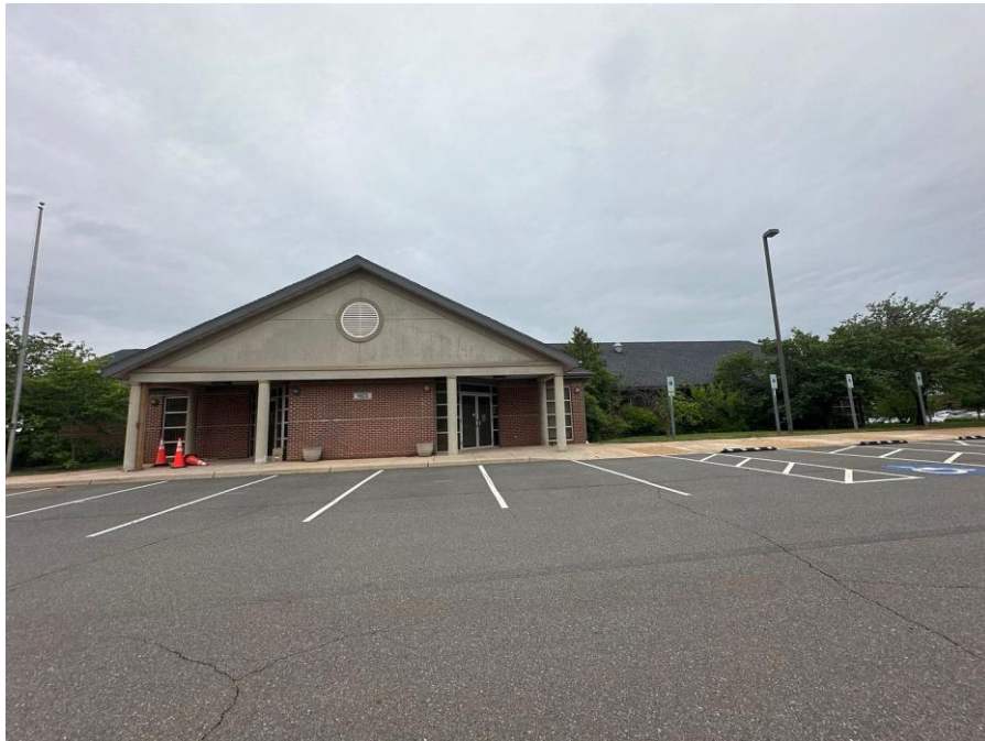
View of Existing Structure
