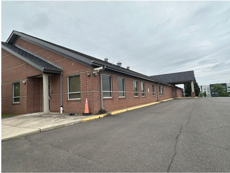
View of Existing Structure
