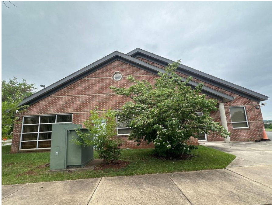
View of Existing Structure
