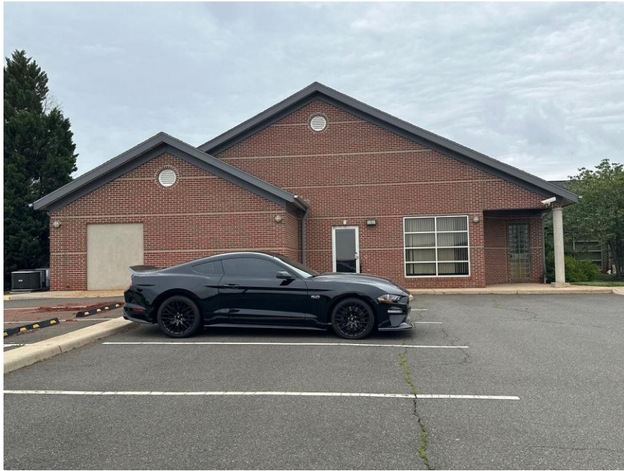
View of Existing Structure
