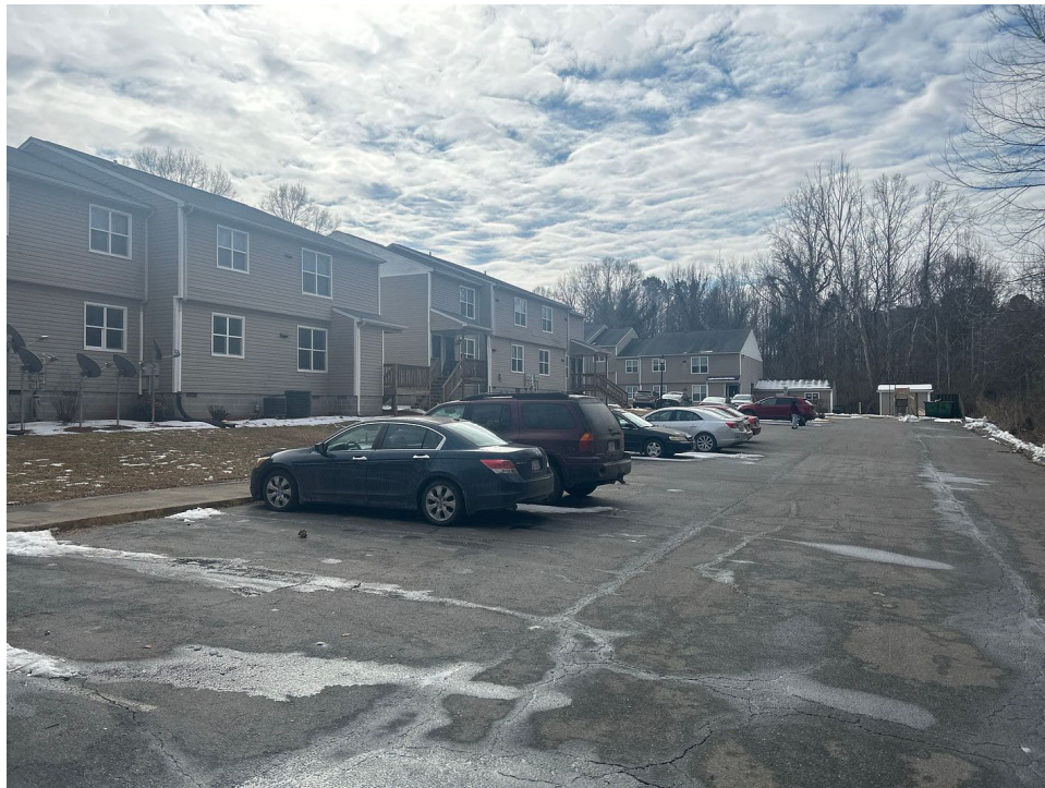
View of Parking
