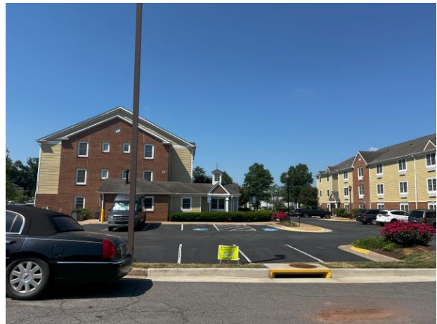
Typical Multifamily Property
