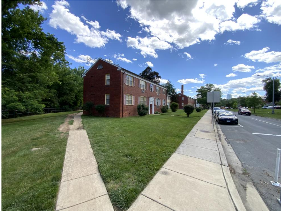
View to the South
