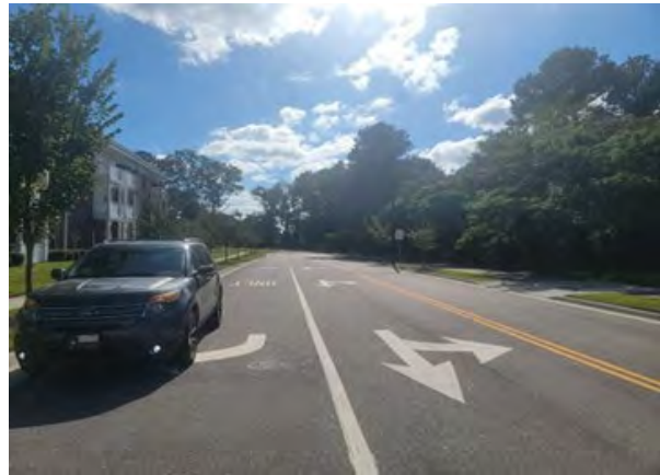
Looking South From Entrance
