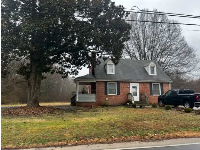
Single-family home west of Subject site
