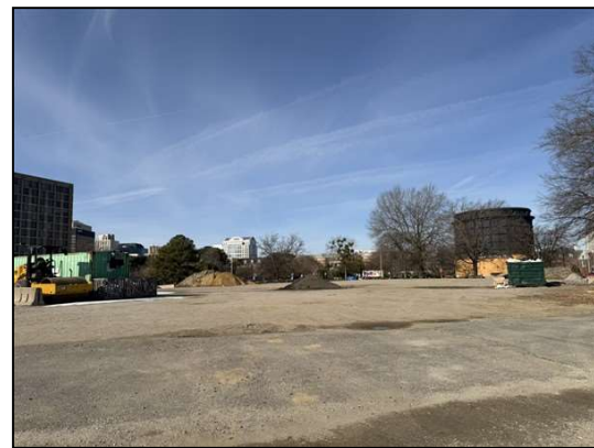
Construction staging site west of site
