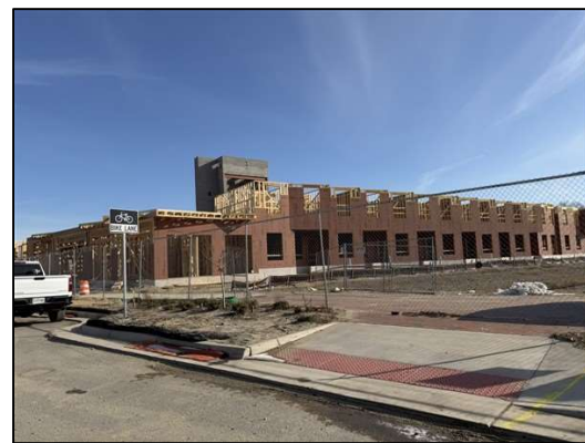
Tidewater Gardens development site north of site
