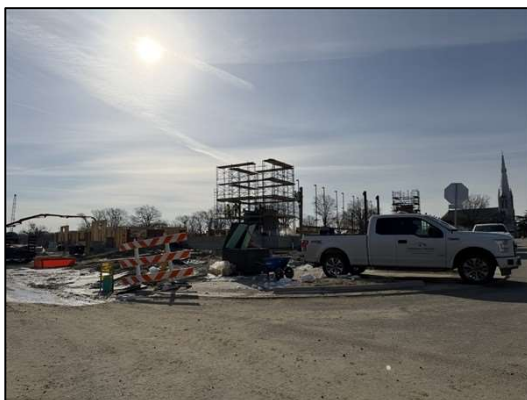
Tidewater Gardens development site north of site
