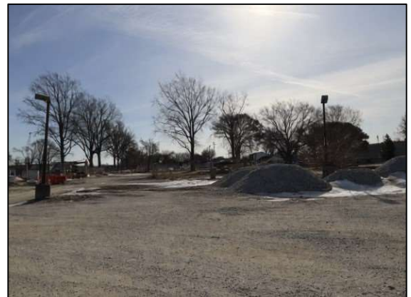
Subject site facing east from Chapel Street
