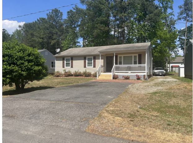
Typical single-family to east
