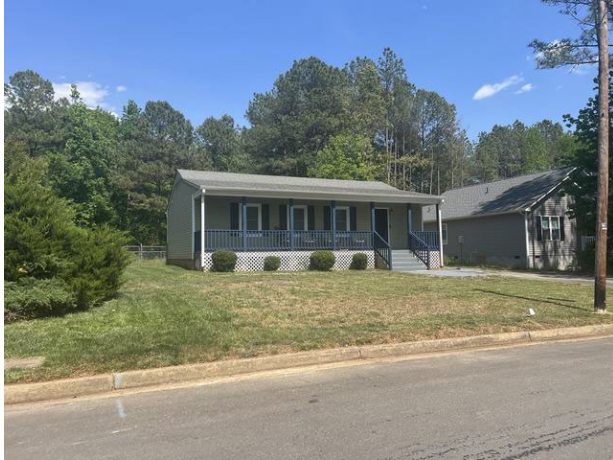
Typical single-family to east
