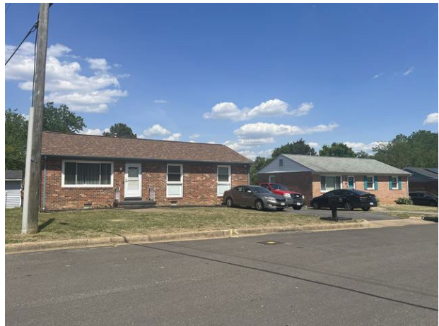
Typical single-family to east
