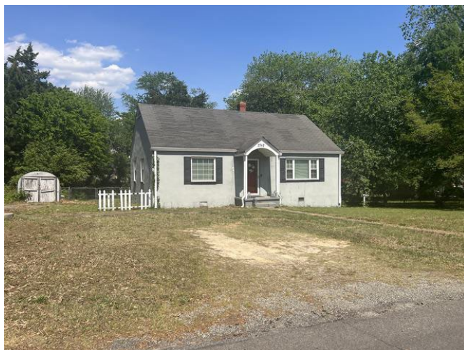
Typical single-family to east
