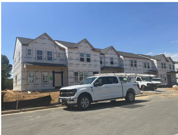
Under construction townhomes to north
