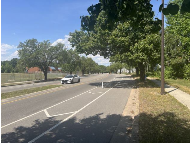
View north along Hopkins Road
