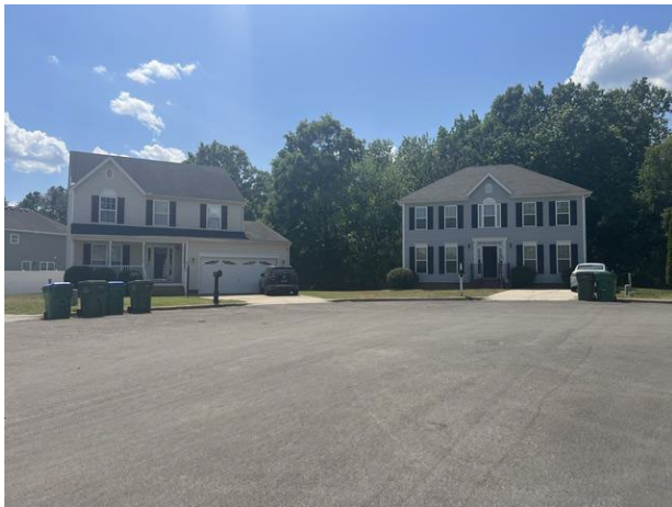
Typical single-family to east
