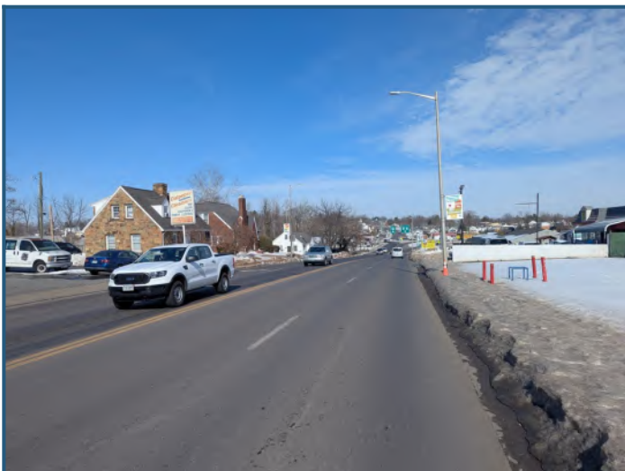
Streetscape: North view of North Main Street
