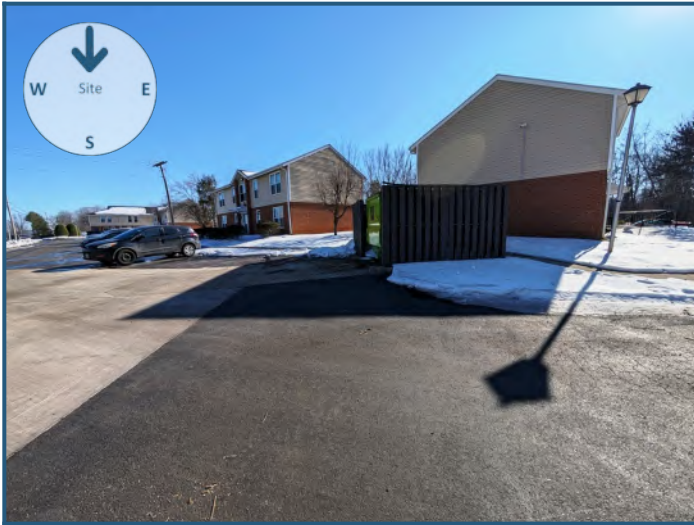
View of site from the north
