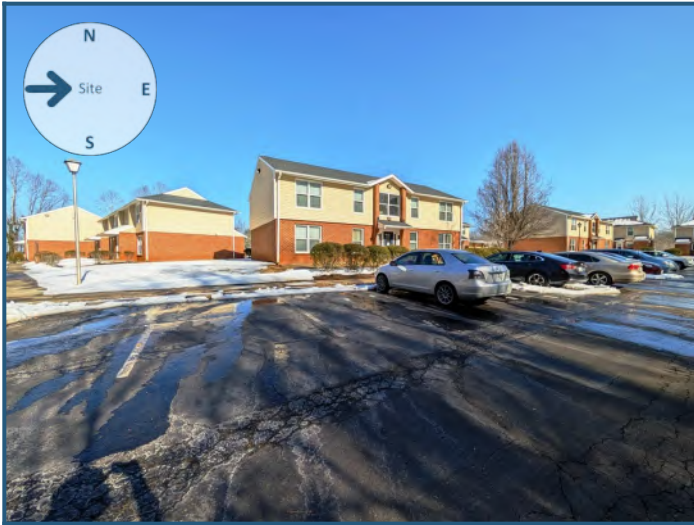
View of site from the west
