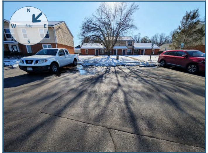
View of site from the northeast
