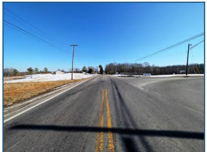
Streetscape: Southeast view of U.S. Highway 60
