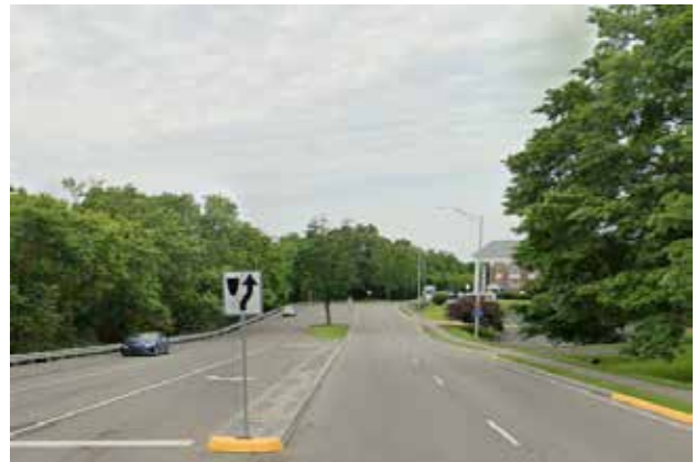
Looking South From Entrance
