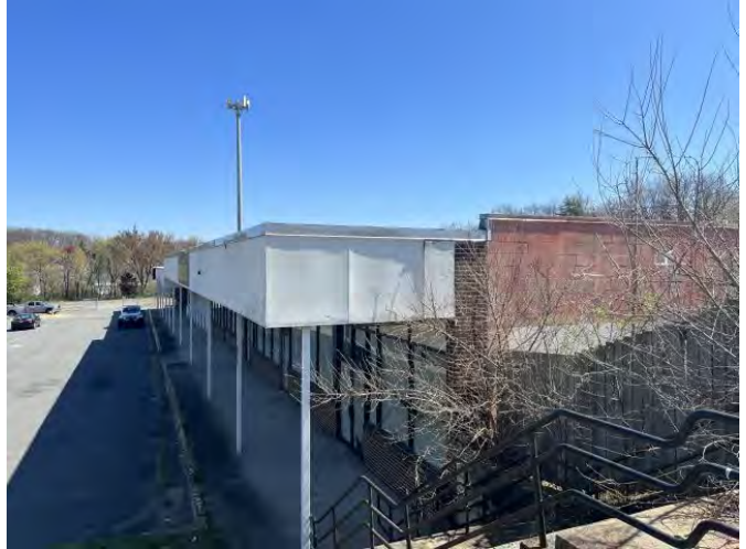
View of the Subject site, existing structures to be razed
