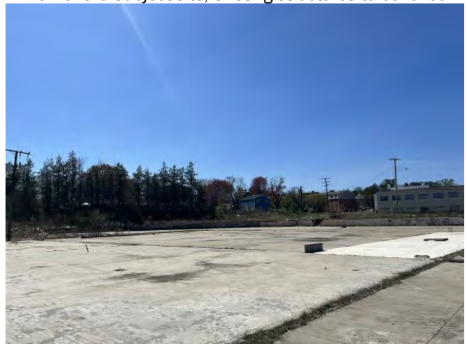
View of parking lot of west side of the Subject site
