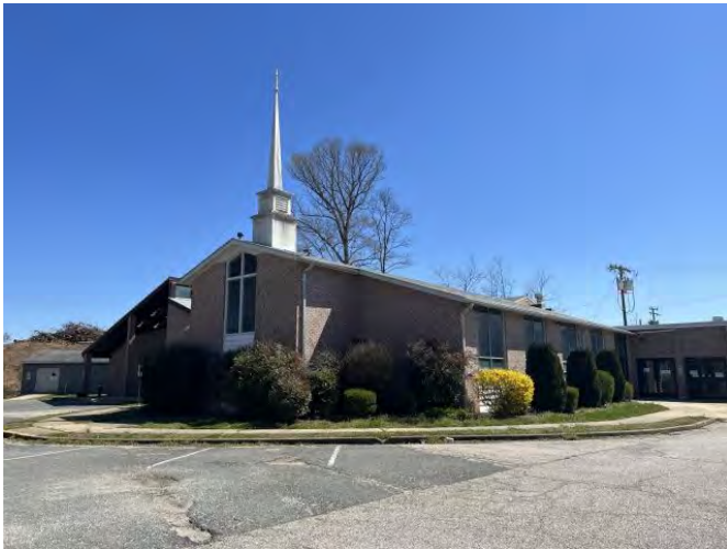
House of Worship northwest of the Subject site
