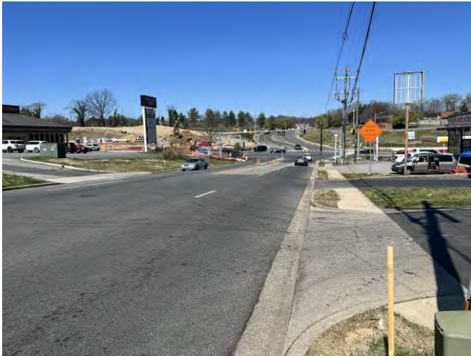
View north along Mt. Pleasant Drive west of the Subject site
