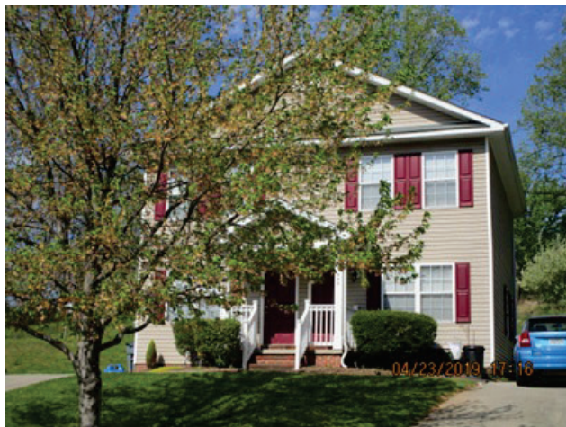
Main Structure Photo
