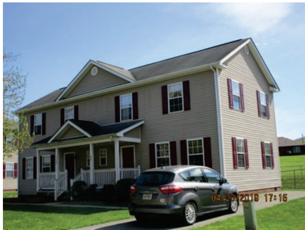
Main Structure Photo
