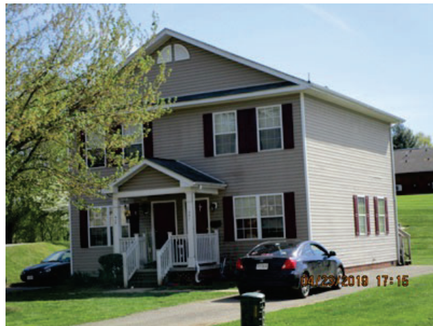
Main Structure Photo
