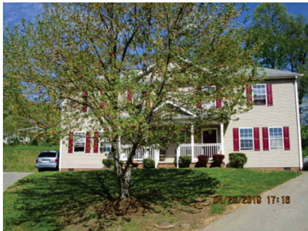
Main Structure Photo
