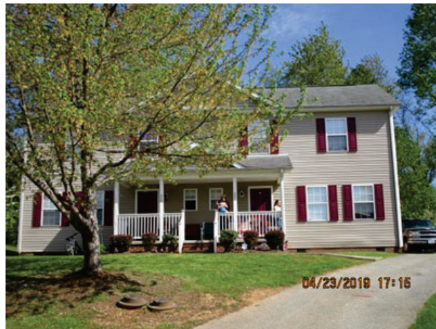
Main Structure Photo
