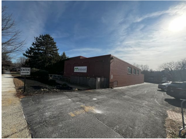
Subject site (existing improvements to be razed)
