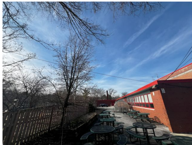
Subject site (existing improvements to be razed)
