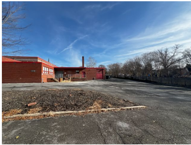
Subject site (existing improvements to be razed)
