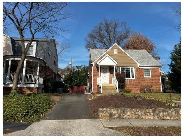
Single-family home north of the Subject site
