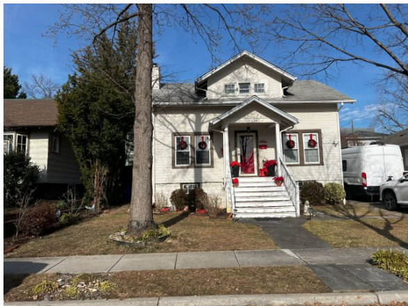
Single-family home north of the Subject site
