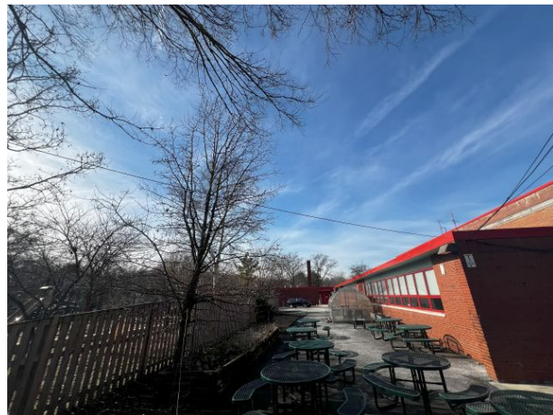
Subject site (existing improvements to be razed)
