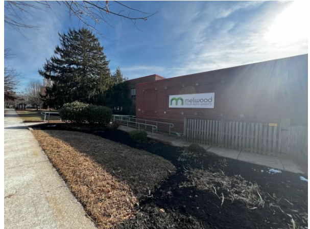
Subject site (existing improvements to be razed)
