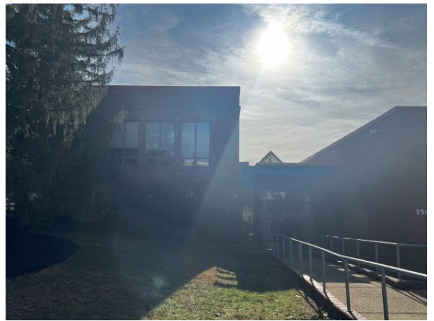
Subject site (existing improvements to be razed)
