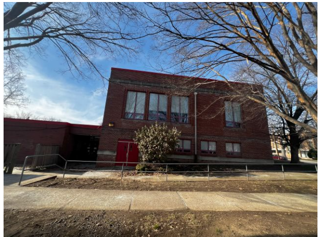
Subject site (existing improvements to be razed)
