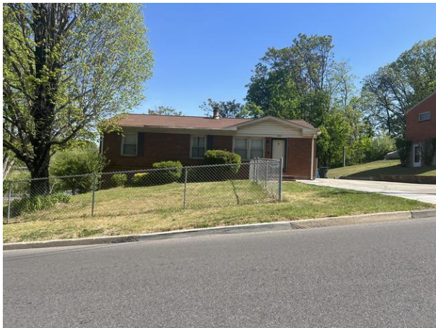
Typical single-family to west
