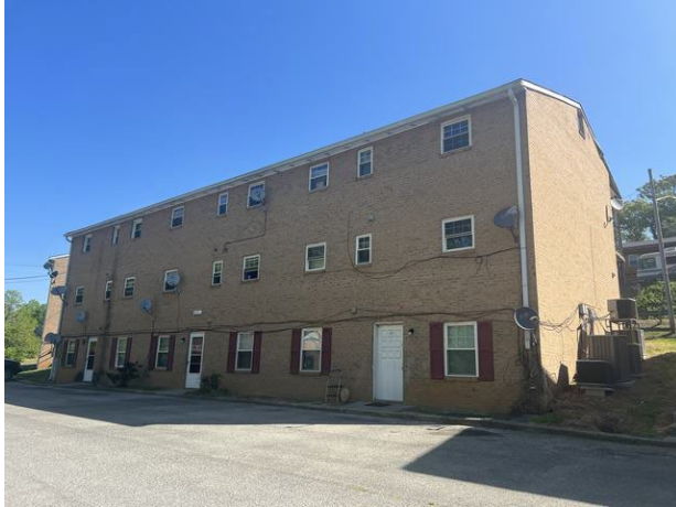
Westside Apartments to south
